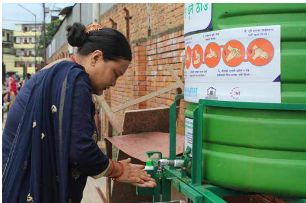
A newly installed touchless handwashing facility by UN-Habitat aims to prevent the spread of COVID-19 in Kalimati Vegetable Market in Kathmandu, Nepal © UN-Habitat Nepal
